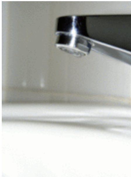
Water dripping from a tap
